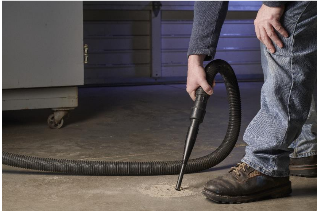
Vacuuming the hole
